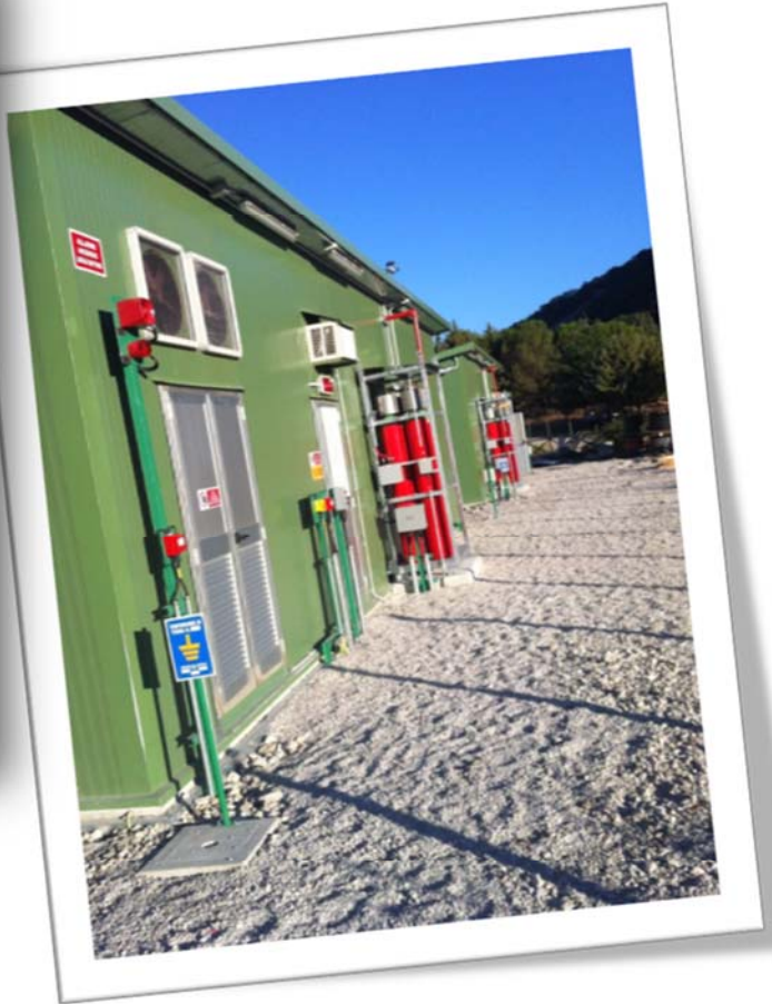
Manufacturing and Installation
